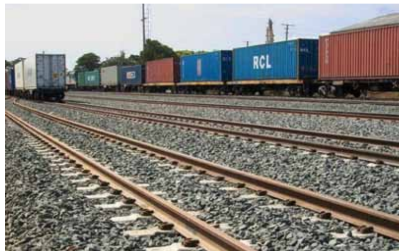
Reconfigured track layout and upgrade works at Port Botany Rail Yard. Photograph courtesy of Australian Rail Track Corporation.
