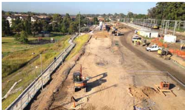
Earthworks for Southern Sydney Freight Line at Liverpool. Photograph courtesy of Australian Rail Track Corporation.
