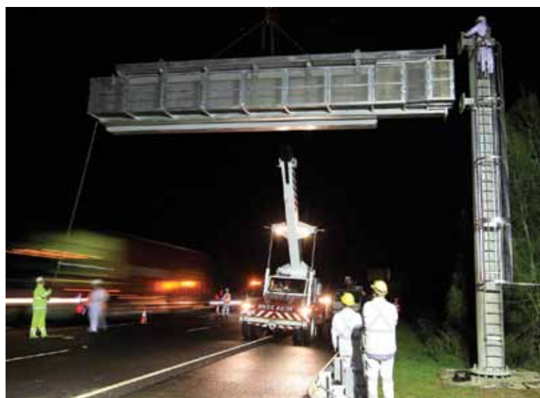
Variable Message Sign Gantry being installed on the M4 west bound near Kingswood road. These signs are for travel times. Photograph courtesy of Roads and Maritime Services, NSW.
